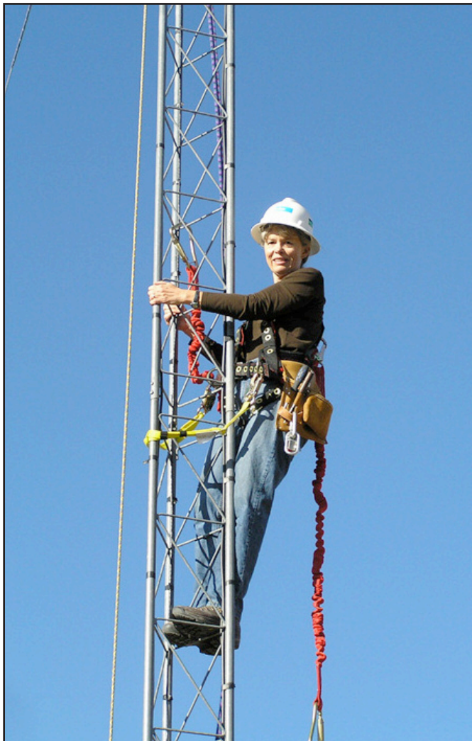
Christine Burke, KØALT, practices using her new fall arrest safety climbing harness on the 69-foot tower at her rural western Colorado station.
