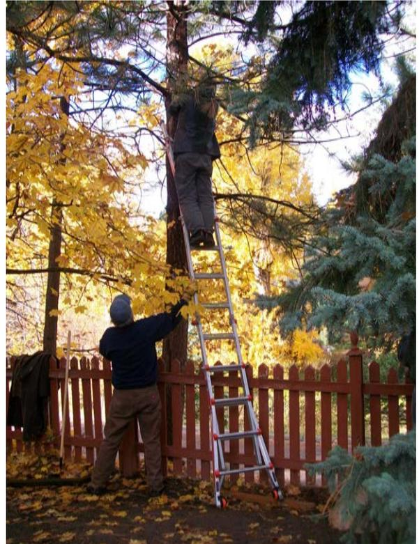
Dick W7XT steadies a ladder while Tom K7QA wraps cable for a pulley in a tree.
